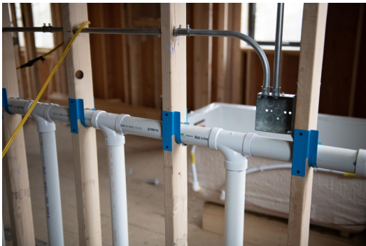
Highly versatile: Secures pipes in a wide variety of locations and positions
