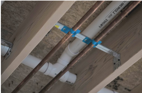
Overhead pipe installation in-between joists and beams
