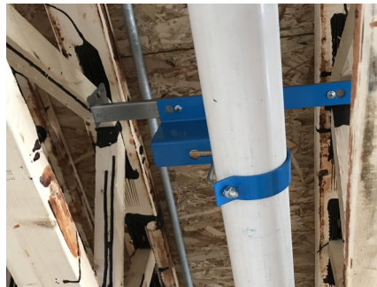
Overhead pipe installation in-between joists and beams
