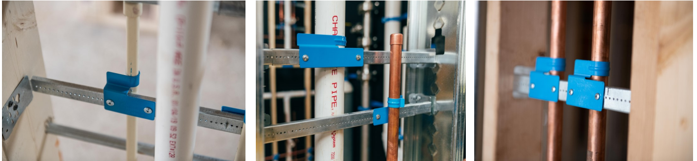
Vertical pipe installation in-between studs
