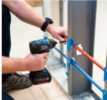
Inside of the wall: Holds and Protects pipes and can be used with both wood or metal studs
