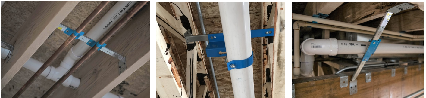
Overhead pipe installation in-between joists and beams
