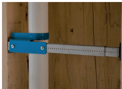
Overhead pipe installation in-between joists and beams
