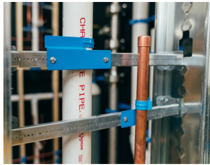
Vertical pipe installation in-between studs
