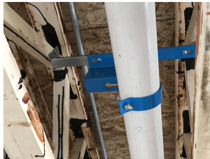
Overhead pipe installation in-between joists and beams
