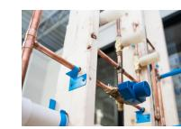
Inside of the wall: For applications that need to go through the center or back of the stud
