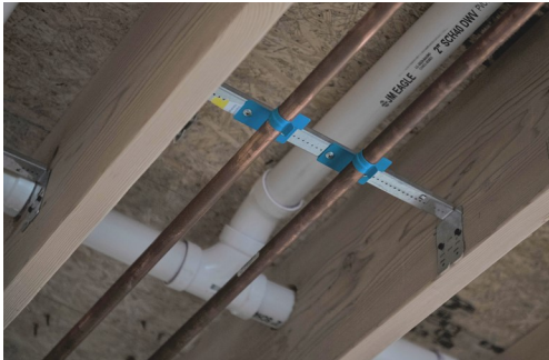
Overhead pipe installation in-between joists and beams
