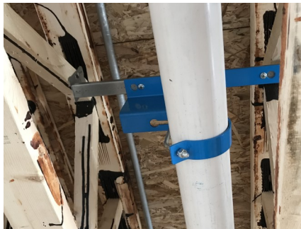
Overhead pipe installation in-between joists and beams
