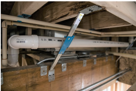
Outside of the wall: For installation applications that need to be mounted on beams or joists
