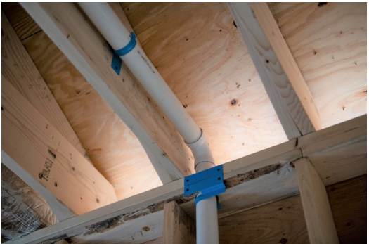
Outside of the wall: For installation applications that need to be mounted on beams or joists
