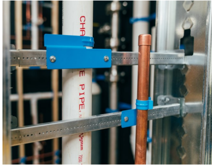
Vertical pipe installation in-between studs
