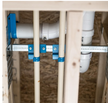
Outside of the wall: For installation applications that need to be mounted on beams or joists
